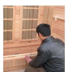
Be careful not to scratch the side panels when positioning the heater panel.
